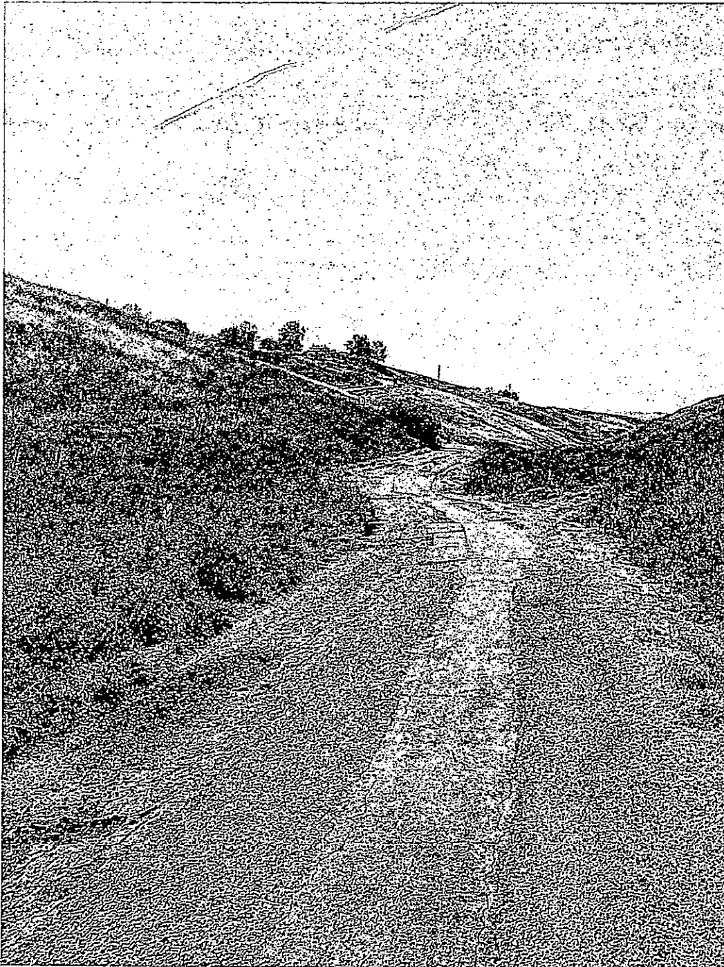
Photo 4: Bald Eagle, Patch Deterioration and Edge Potholes
