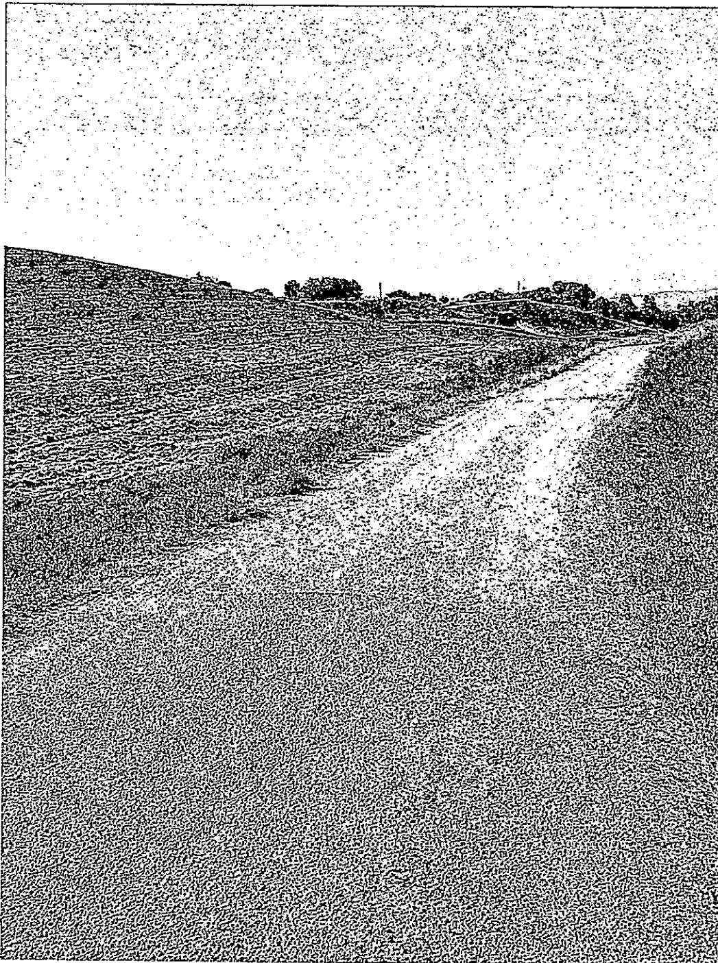
Photo 7: Ojas Azules Place, Gravel/Chip Seal Boundary with Minor Rutting
